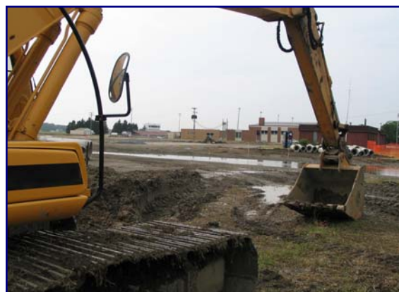
Otsego High School - Under Construction
