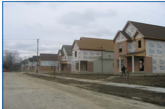
City West Village Under Construction
