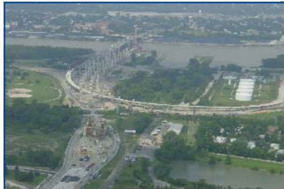
Construction of the Cable-Stayed I-280 Bridge
